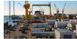
An improved automated process of scheduling and assignment of build unit lay-down locations can result in a significant savings at the highly functioning Ingalls Shipyard.
